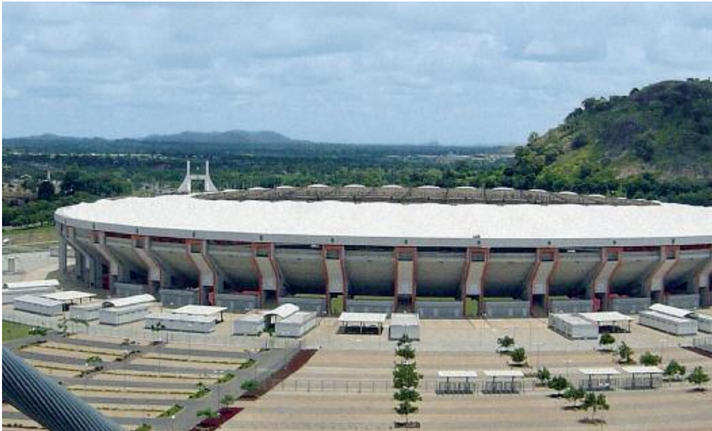
The floodlighting at Abuja Stadium in Nigeria is controlled entirely by GAMMA instabus .
