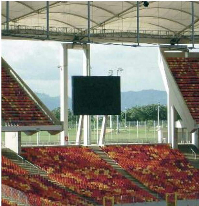
Flood-light operation at Abuja Stadium in Nigeria with GAMMA instabus .
