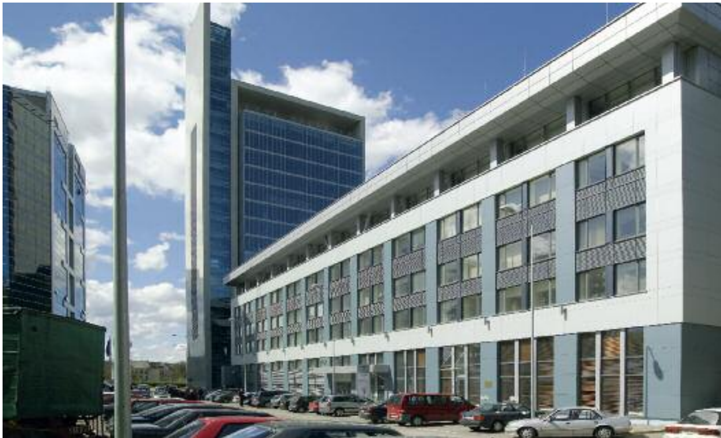
This modern, six-story office building in Vilnius, Lithuania, is also the home of the Siemens Lithuania Head Office.
