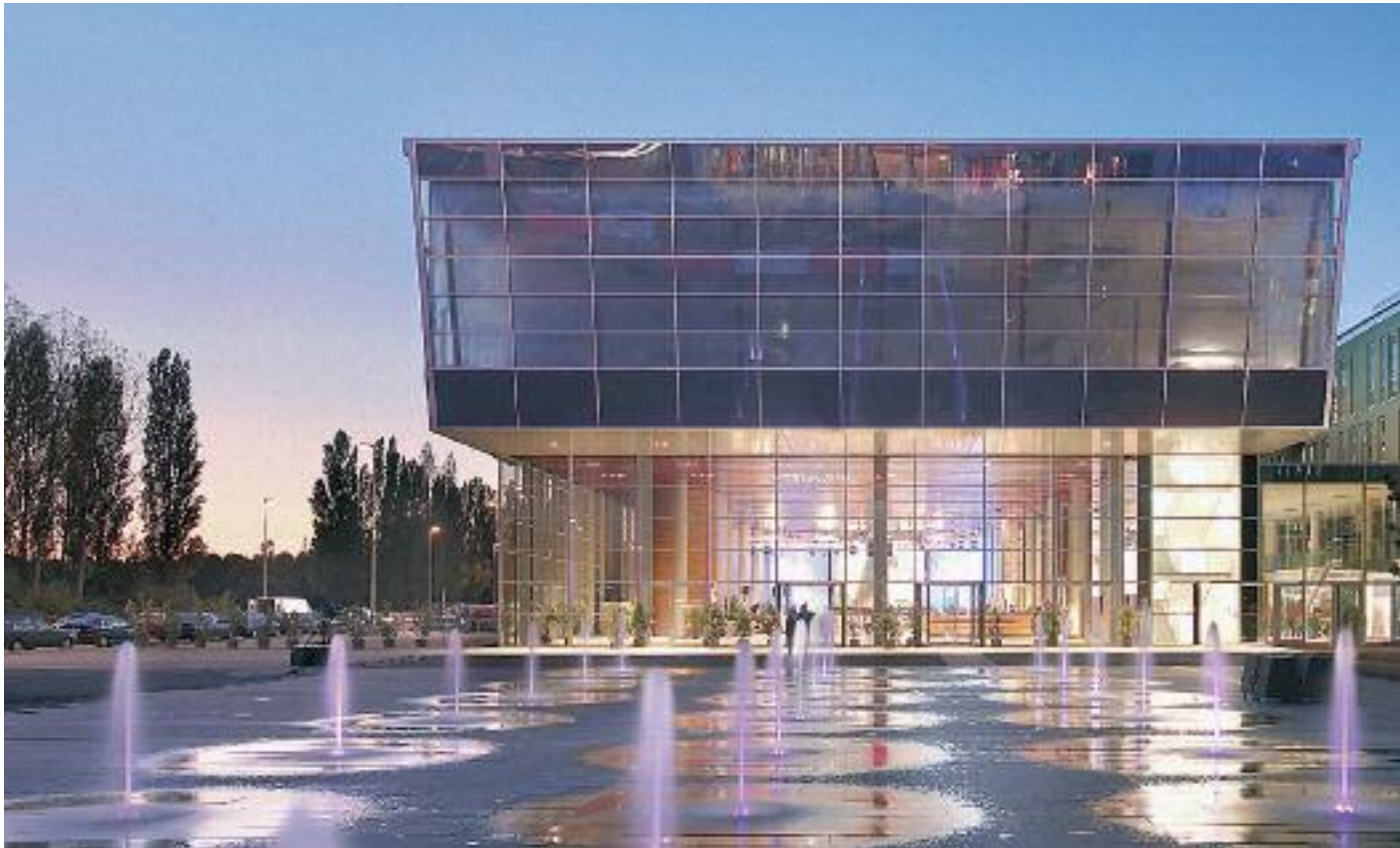
Efficient GAMMA instabus technology blends harmoniously with ambitious architecture at the Head Office of T-Mobile in Bonn.
