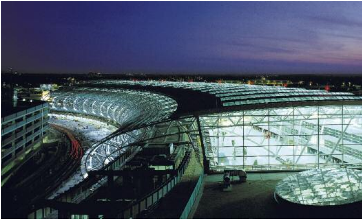
Duesseldorf Airport trusts in a future-proof building management system from Siemens.
