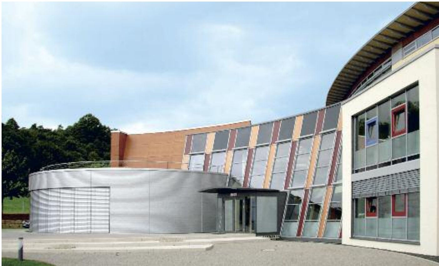
Individual and comfortable building management provided by GAMMA instabus at NICI AG.
